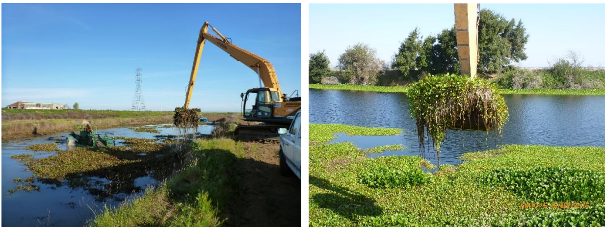
Photos: Surface excavator removal (DBW).
