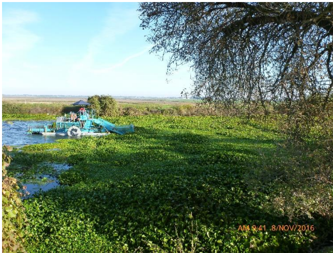
Photo: Mechanical cutter and conveyor equipment being used on water hyacinth (DBW).
